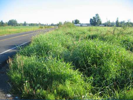
Looking north on 244Ave SE. This used to be a clear 5-6' deep ditch to handle the rainy season. WA State and King Country environmental pandering insanity ignores this until it floods over the intersection. Then they propose another green taking, a $500,000 concrete fish roundabout.
